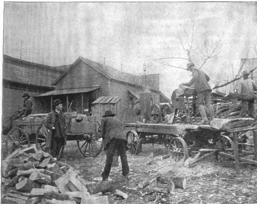
A PORTABLE WOOD-SAWING OUTFIT DRIVEN BY A GASOLINE ENGINE.
