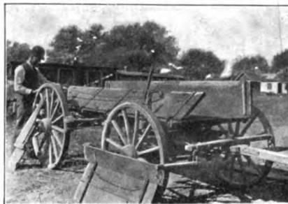
Fig. 2. THE SIDE BOARDS—METHOD OF FASTENING.
