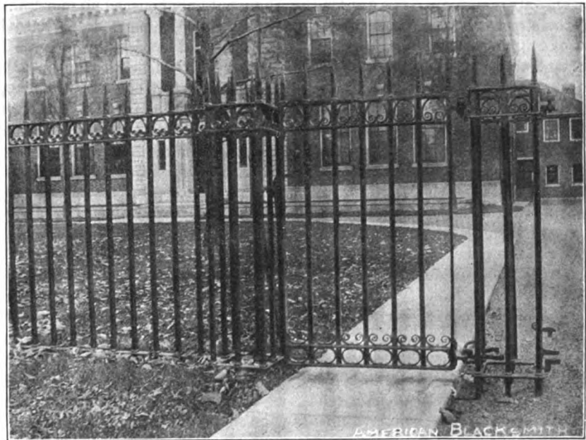
A NEAT, PLAIN STYLE OF WROUGHT IRON FENCE.
