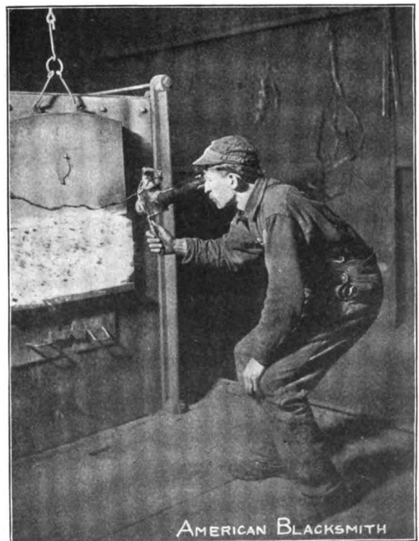
FIG. 3. TAKING FURNACE TEMPERATURES.
