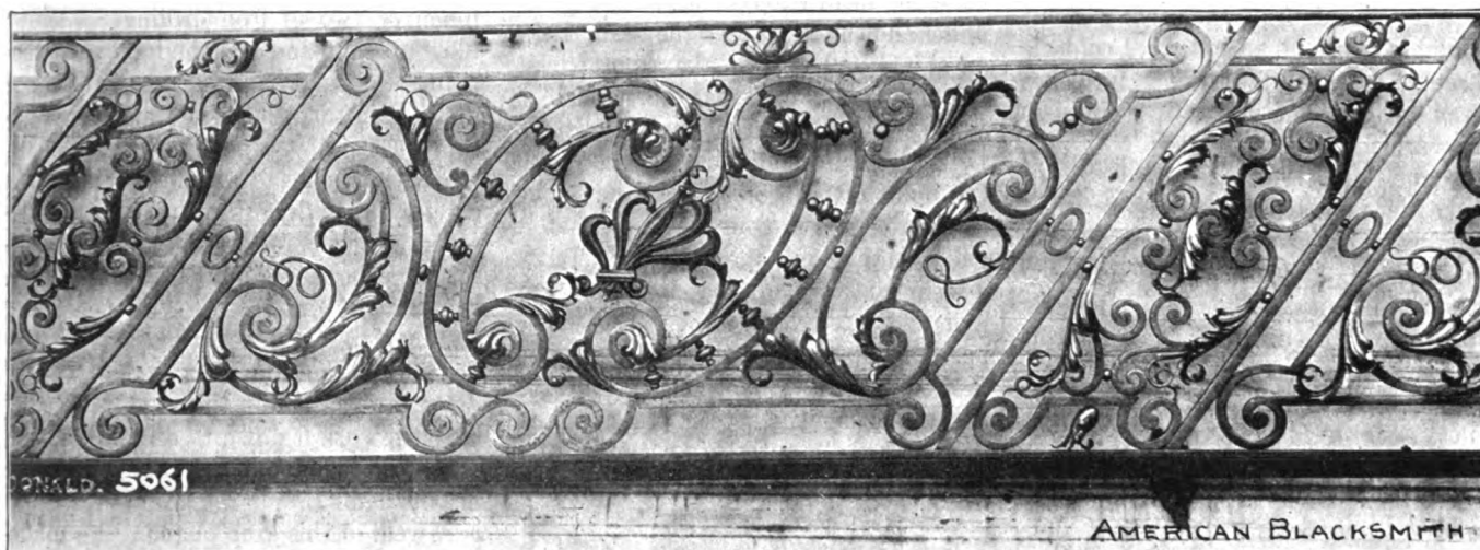
DIAGONAL SCHEME FOR ORNAMENTAL IRON STAIR RAILING
