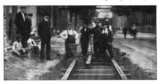
OUTFIT AND METHOD USED IN WELDING RAILS WITH THERMIT. TIME REQUIRED FOR EACH WELD, FROM THE PREPARATION OF JOINT TO COMPLETION OF OPERATION, TEN MINUTES.
