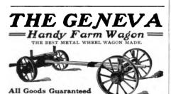
Pressed steel wheels, any height and width tire, interchangeable hubs. Gears of selected stock, thoroughy ironed. Made in several styles.
