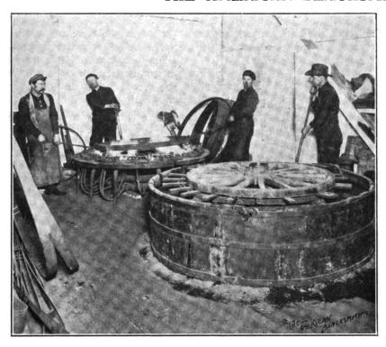
ANOTHER VIEW OF THE WAGON REPAIRING DEPARTMENT SHOWING GAS TIRE HEATER IN OPERATION.
