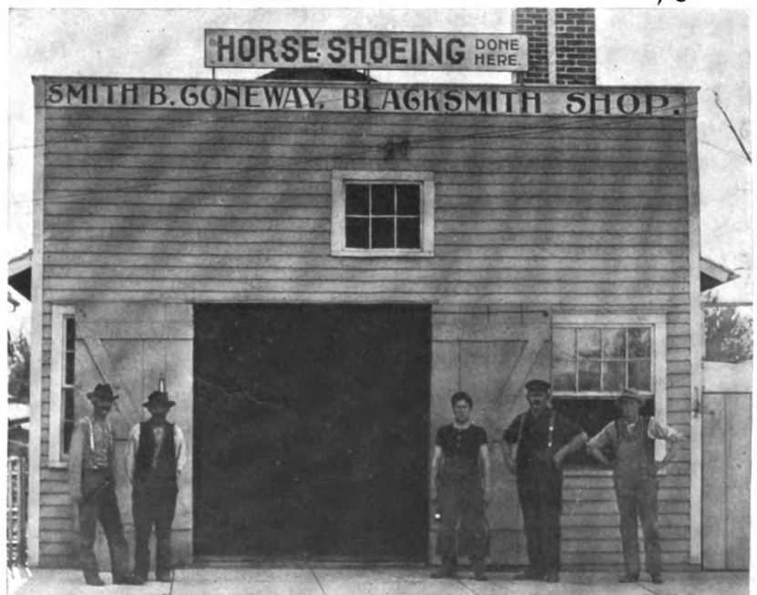
A GENERAL SHOP OF INDIANA WHOSE OWNER HAS SEEN HALF A CENTURY OF SERVICE BESIDE THE FORGE
