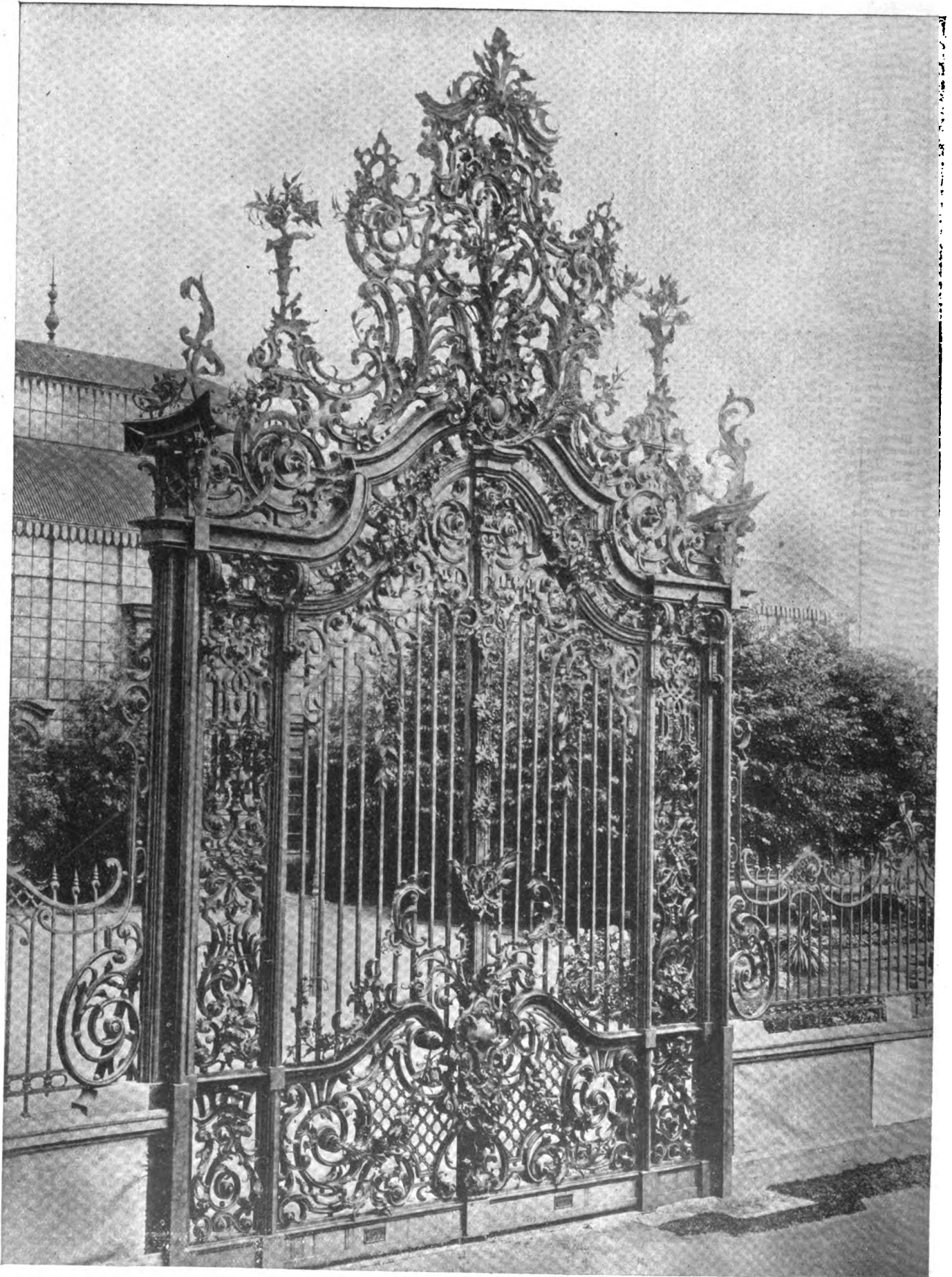
AN EXQUISITE EXAMPLE OF HAND-WROUGHT WORK FROM THE FORGES OF ARMBRUSTER BROTHERS OF GERMANY. THIS IS ONE OF THE MANY SIMILAR GATES THAT LEAD TO THE GROUNDS SURROUNDING THE GERMAN EMPEROR'S PALACE AT POTSDAM
