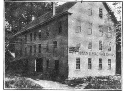
FOR THE REPAIR OF THE HORSELESS VEHICLE
