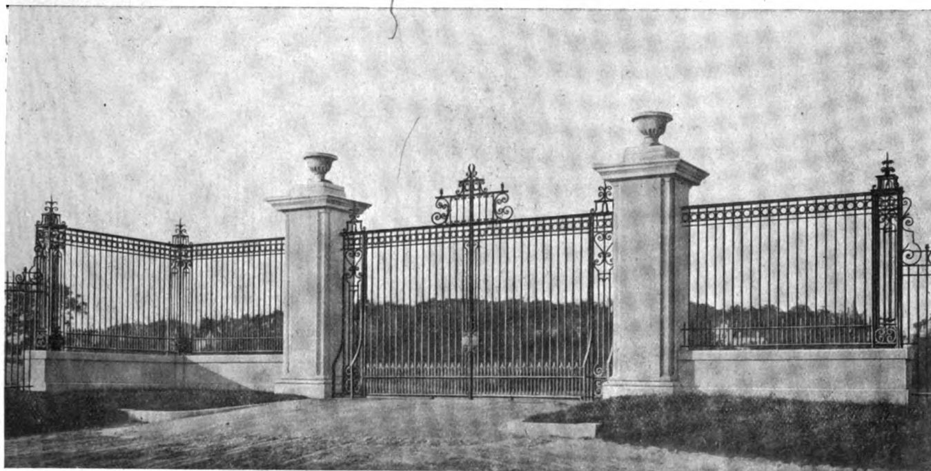
SIMPLICITY AND DIGNITY OF DESIGN COMBINE TO MAKE THIS ENTRANCE GATE AN EXCELLENT ONE FOR A CEMETERY
