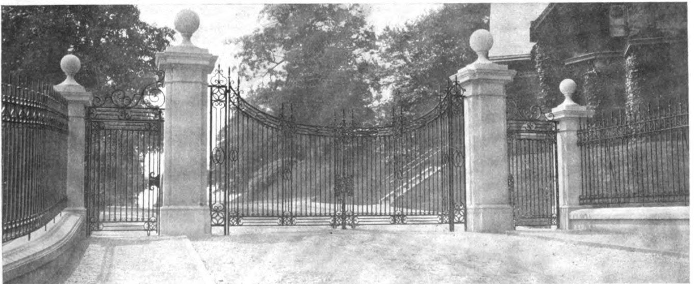
A VERY GRACEFULLY DESIGNED GATE PLEASINGLY FREE FROM OVER ORNAMENTATION. IT ACCORDS WELL WITH ITS SURROUNDINGS
