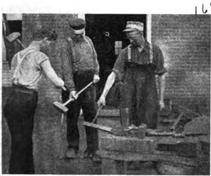
FIG. 1.—THE CRANK IS HELD FIRMLY WHILE BEING WELDED
