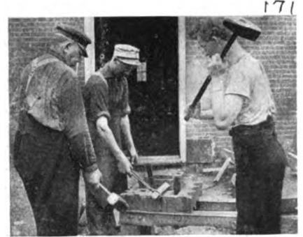
FIG. 2.—ANGLE IRONS CAN BE BENT CONVENIENTLY
