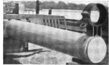
THE CAP BAND AS IT APPEARED ON THE MAST
