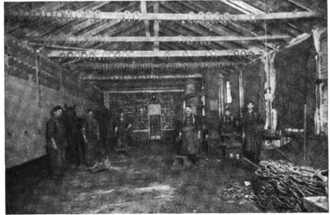
INTERIOR OF PROFESSOR RICH'S SHOP, SHOWING SHOES ON REAR WALL
