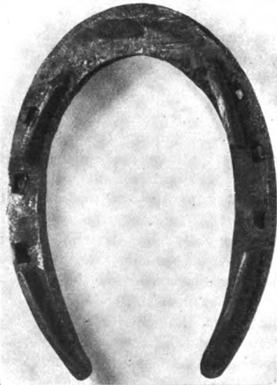
FIG. 2—A SHOE WITH FOUR TAPERED CALKS
