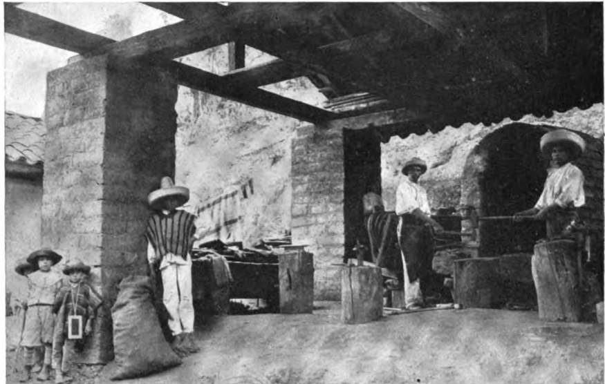
A MODEL MEXICAN SMITH SHOP, WITH ITS ANVILS OF RAILROAD RAIL, ITS PRIMITIVE BELLWS, AND ITS VISE FROM "THE STATES"
