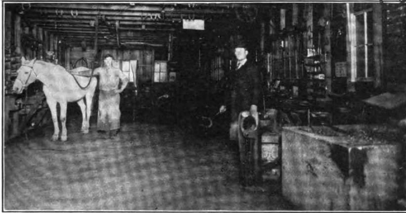
A VIEW OF THE SHORING DEPARTMENT IN MR. ARMSTRONG'S SHOP
