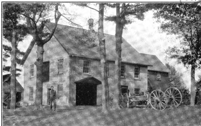
A MODERN CONCRETE SHOP OF ONTARIO, CANADA. MR. W. J. LILLICRAP DOES GENERAL WORK, WOODWORK, AND PAINTING
