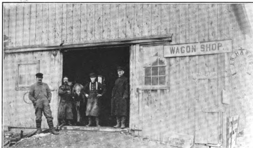
AN EXTERIOR VIEW OF MR. J. B. HARRIS'S GENERAL SMITH SHOP
