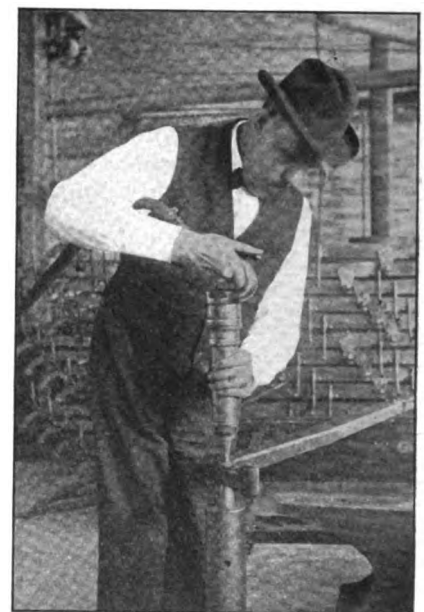
FIG. 2.—A RIVETING HAMMER IN OPERATION
