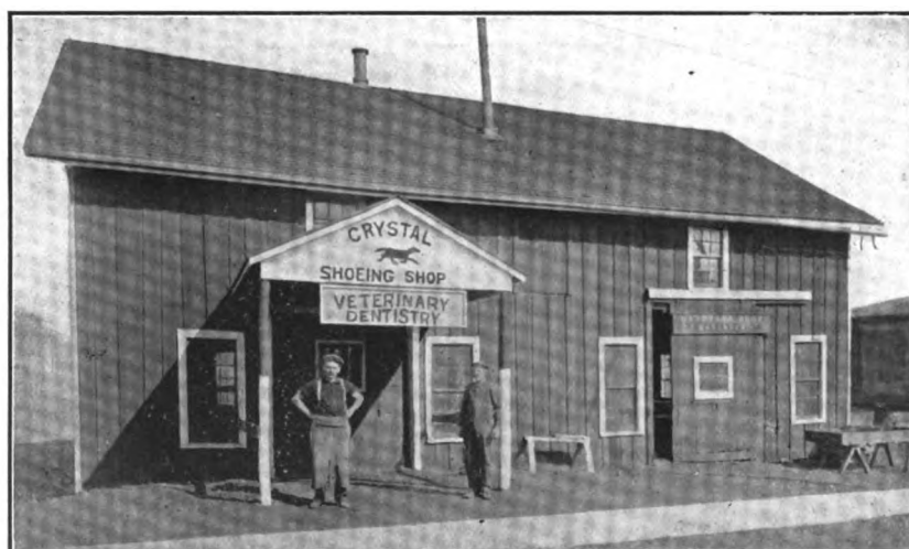
AN EXTERIOR VIEW OF MR. STACY'S SHOEOING SHOP. THE INTERIOR IS SHOWN IN THE FRONTISPIECE
