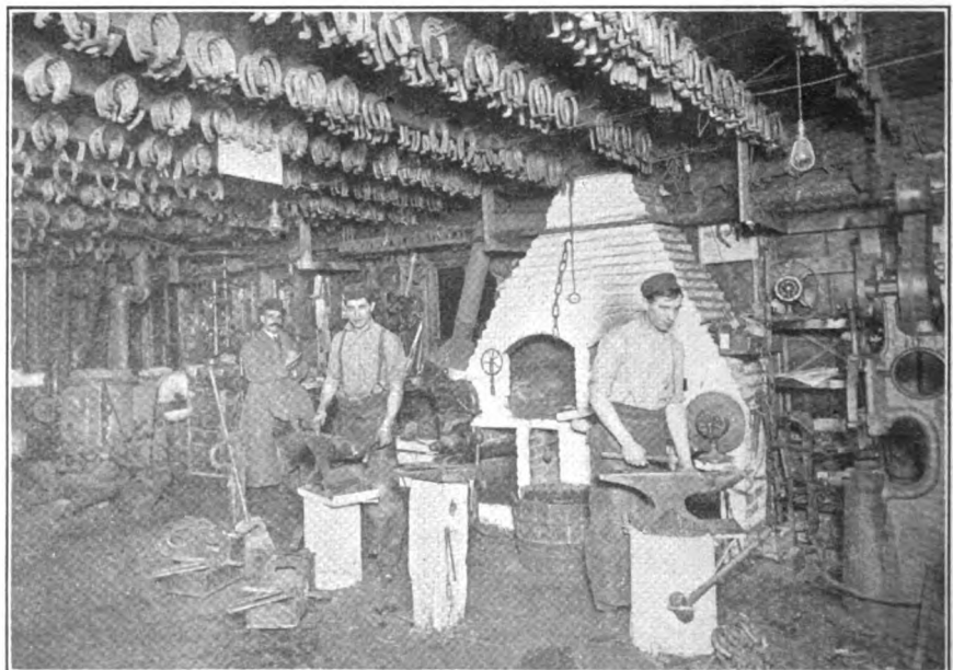
AN ILLINOIS SHOP USING ELECTRICITY FOR BOTH POWER AND LIGHT
