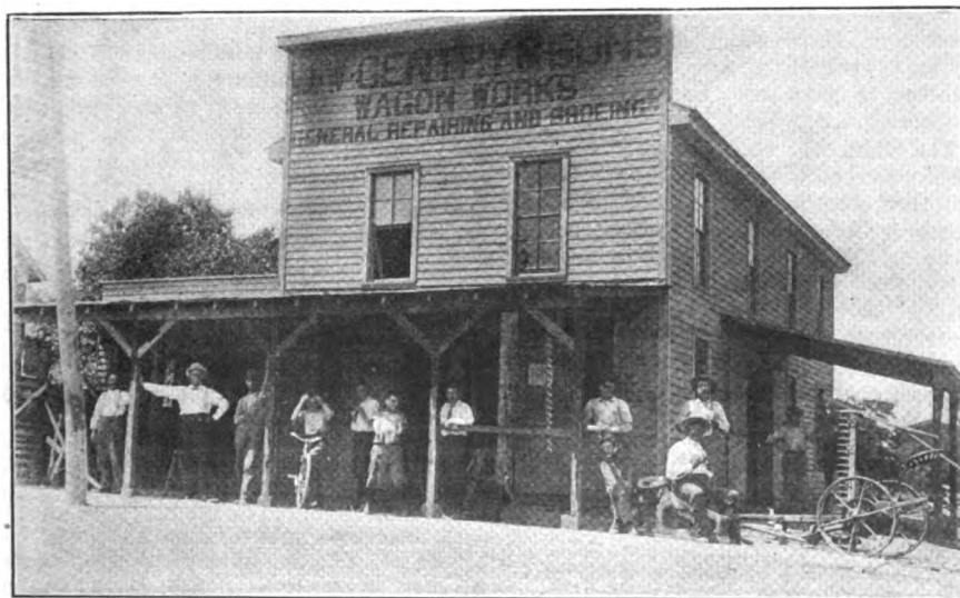
THIS KENTUCKY SHOP IS WELL EQUIPPED WITH POWER MACHINES
