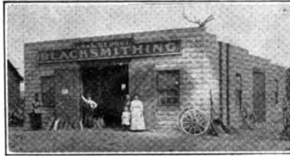
A WYOMING SMITHY OF CONCRETE OPERATED BY MR. CHARLES GEORGE
