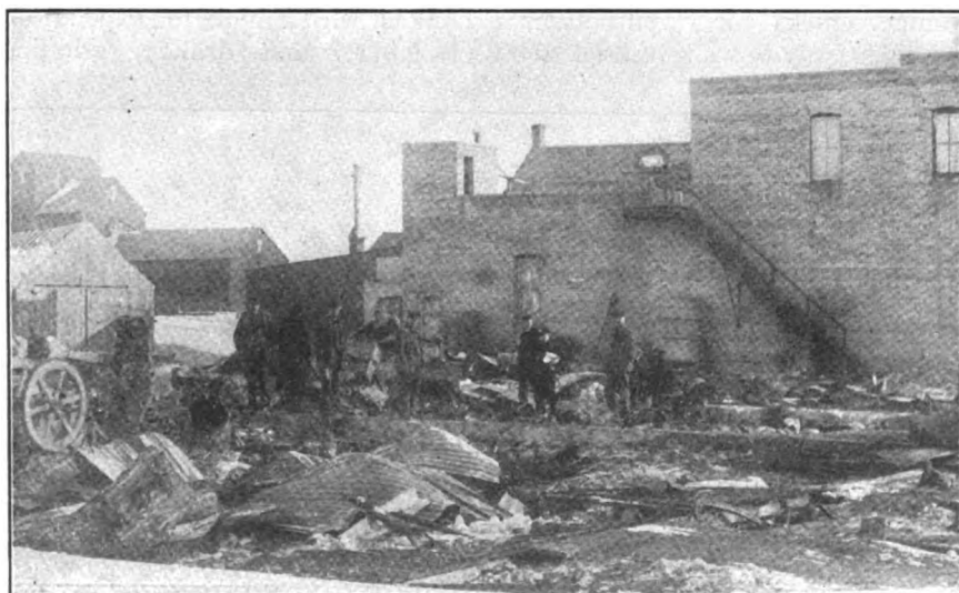
AFTER THE FIRE—WHAT WAS LEFT OF MR. NELSON'S SHOP AND POWER EQUIPMENT
