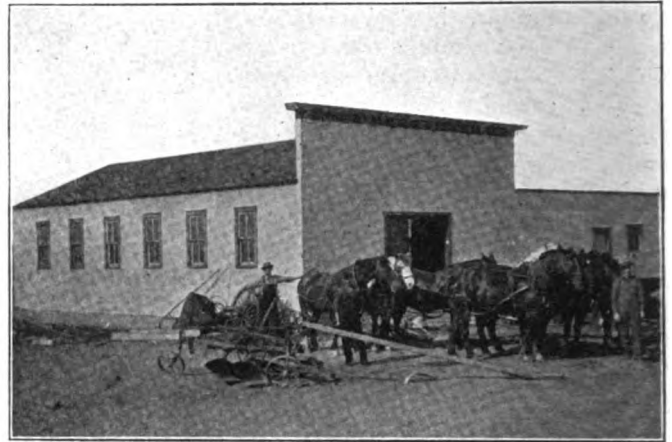
THE PRESENT SHOP OCCUPIED BY WOLD BROS. WAS BUILT LAST FALL
