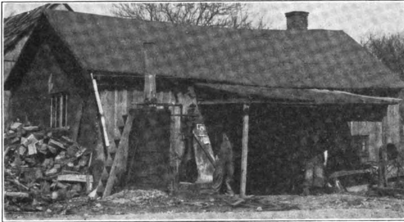
THE OLD SHOP OF THARP & SPANGLER. NO ROOM INSIDE FOR THE POWER PLANT
