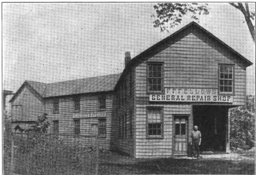
A WELL-BUILT GENERAL SMITHING AND WOOD-WORKING SHOP OF NEW YORK STATE
