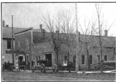
THE WISCONSIN GENERAL SHOP AND CONCRETE GARAGE OF MR. O. G. KLEIN
