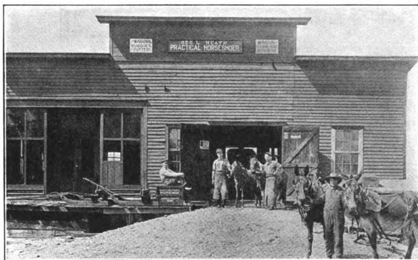
THE POWER SHOP OF MR. GEORGE L. HEATH OF PENNSYLVANIA
