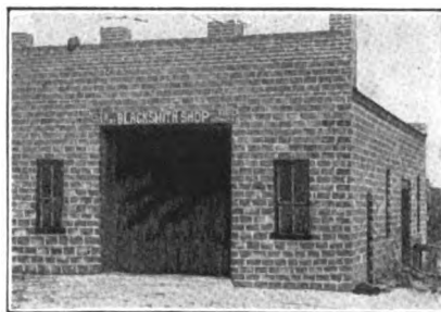
A WELL-BUILT SHOP OF HOLLOW TILE CONSTRUCTION
