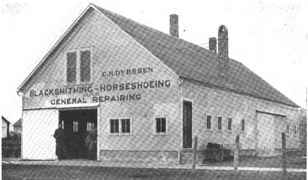
THE PRESENT SHOP OF MR. DYRSSEN IS WELL EQUIPPED WITH MACHINES
