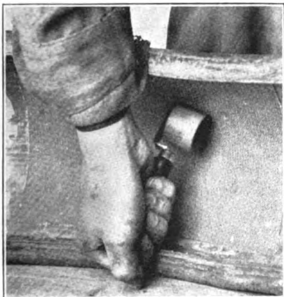
FIG. 6—HOW THE PATCHES ARE APPLIED AND ROLLED INTO PLACE
