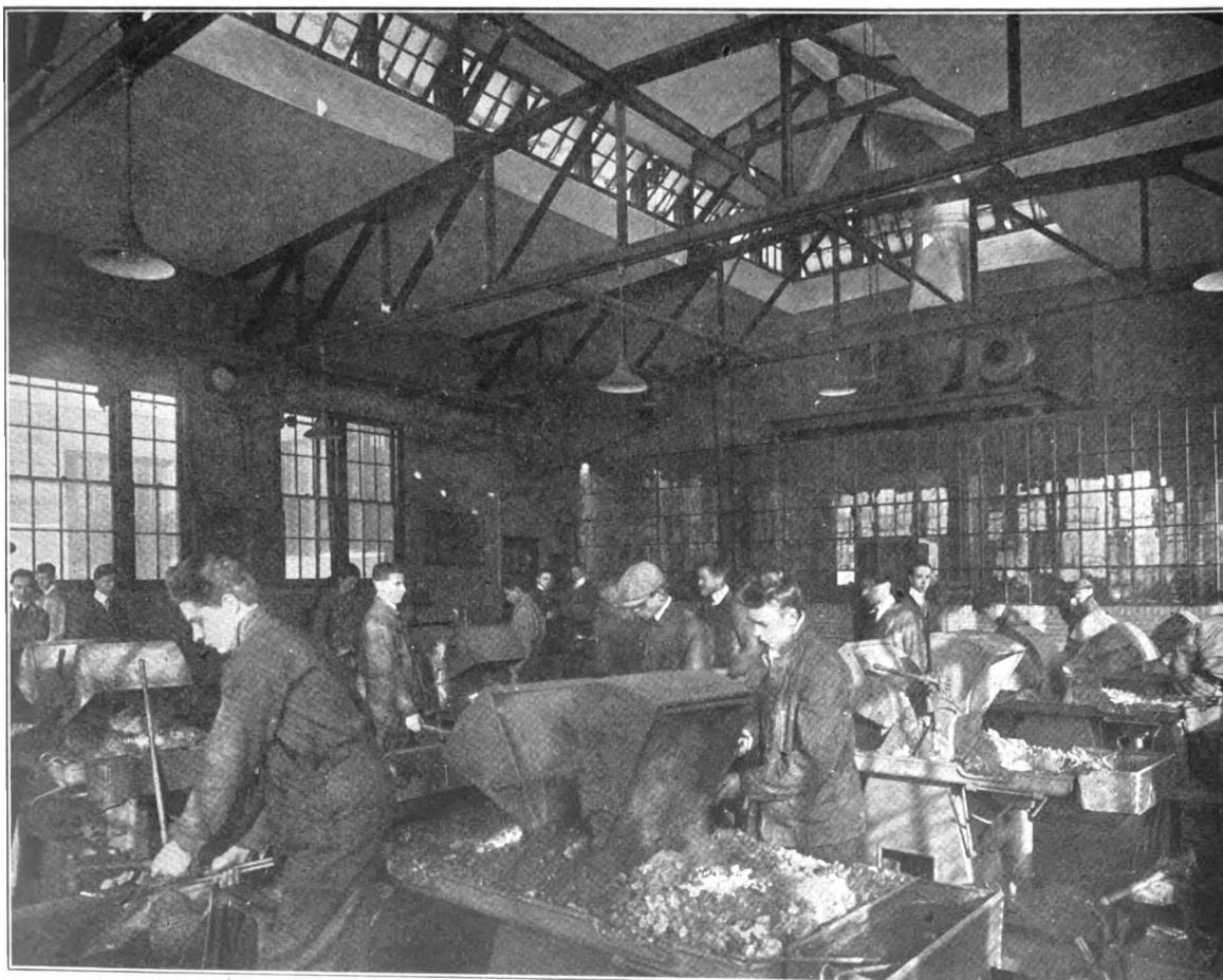
A BATTERY OF TWENTY-FIVE MODERN DOWN DRAFT FORGES COMPRISE THE PRINCIPLE FORGE SHOP EQUIPMENT
