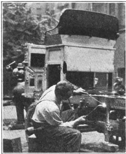
FIG. 8—HERE A THREE-TON TRUCK FRAME IS BEING WELDED
