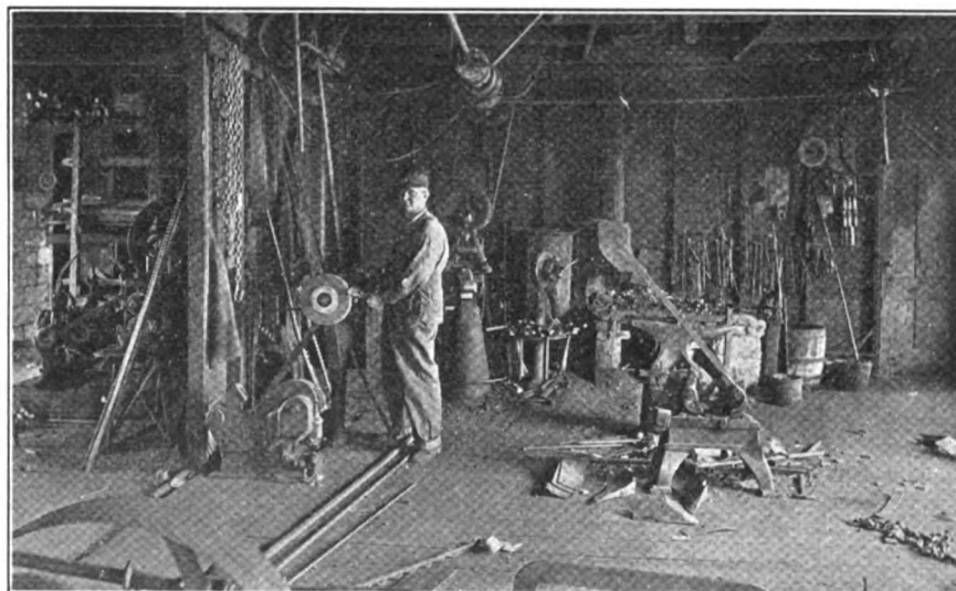
MR. A. E. HAIDY'S KANSAS SHOP IS FULLY EQUIPPED WITH POWER TOOLS AND AN OXY-ACETYLENE MACHINE
