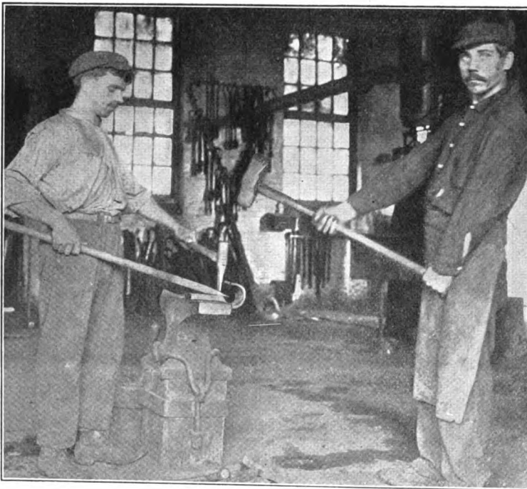
FIG. 3.—HOW ANOTHER LITTLE SAFETY DEVICE SAVES THE HELPER AND OTHER WORKMEN
