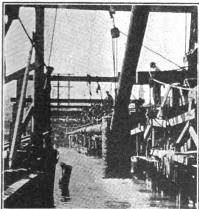
FIG. 5.—READY TO BE SUNK TO THE BOTTOM
