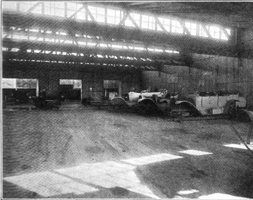
ONE OF THE SPACIOUS SHOPS OF MR. ALBRIGHT'S UP-TO-DATE PLANT. NOTE THE "SAW-TOOTH" CONSTRUCTION OF THE ROOF.
