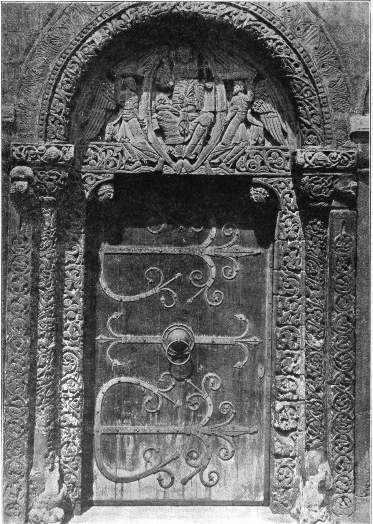
FINE EXAMPLE OF NORMAN WROUGHT IRON WORK ON THE DOOR OF WOKING CHURCH
