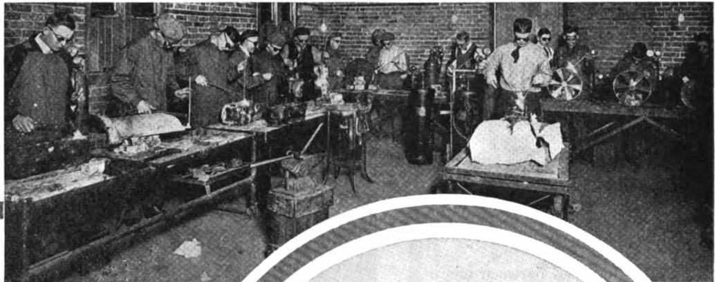
CLASS IN BRAZING, WELDING AND CUT- TING—LEARNING BY DOING
