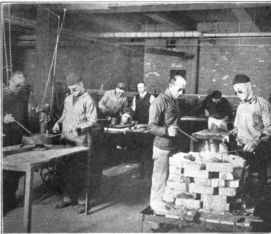
WELDING WITH THE OXY-ACETYLENE FLAME ON TABLES MADE BY THE MEN. THE BRICKS ON THE RIGHT ENCLOSE A FIRE WHICH IS BUILT AROUND A LARGE CYLINDER BEING REPAIRED
