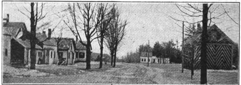
MR. ARTHUR A. BURNAP'S ESTABLISHMENT IN NEW HAMPSHIRE, THE BLACKSMITH, AUTO REPAIR SHOP, PAINT SHOP AND OFFICE ARE ON THE LEFT. THE BUILDING WITH THE GLORIFIED BARBER SHOP EFFECT AT THE RIGHT IS HIS WAREHOUSE.
