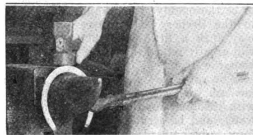
Fig. 18—Shaping the shoe when too narrow at toe.
