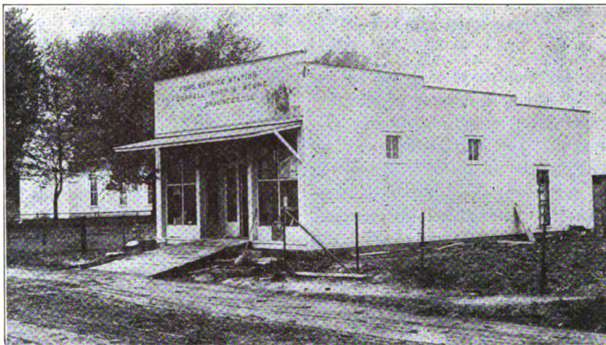
There's nothing particularly impressive about this shop and store as a piece of architecture but Fred's motto above shows one reason why it is one of the best known establishments in rural Illinois—the other reason is Fred himself
