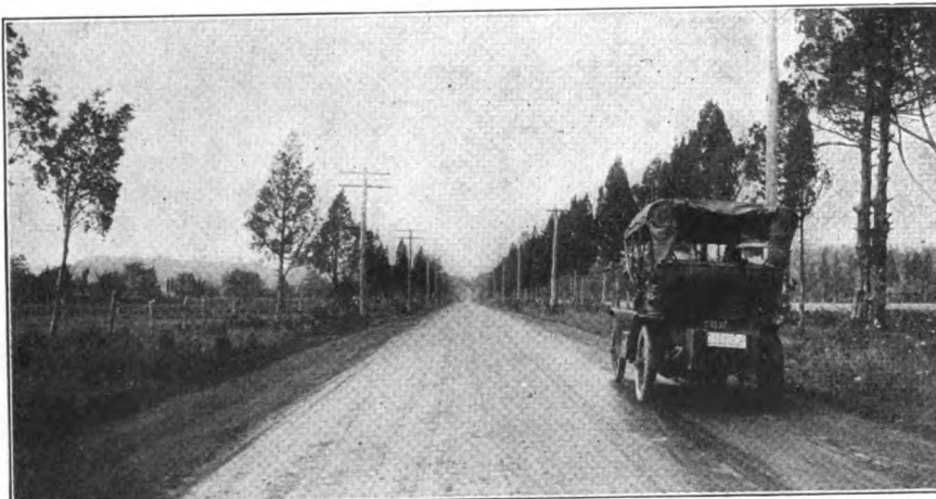
NO MATTER HOW FAST THE AUTOMOBILE GOES IT CANNOT EXTRACT THE BONDING DUST FROM A ROAD LIKE THIS, WHICH IS A PROPERLY BUILT ASPHALTIC, OR BITUMINIZED MACADAM HIGHWAY
