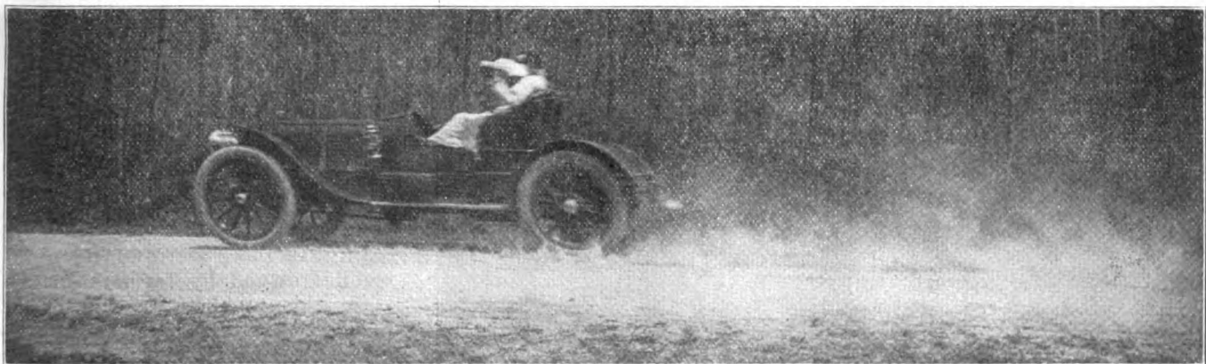
AN EXAMPLE OF THE HARM DONE TO A MACADAM ROAD BY AUTOMOBILE TRAFFIC. NOTE THE SUCKING ACTION OF THE WHEELS IN PULLING THE BONDING DUST FROM THE STONE ROAD. THE WIND CARRIES THIS DUST TO THE ROADSIDE AND DEPOSITS IT WHERE IT IS VALUELESS TO THE ROAD ITSELF.
