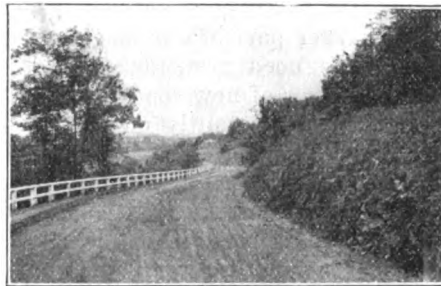
WELL BUILT MACADAM
