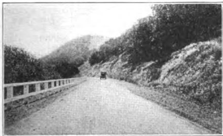
BRICK ROAD COVERED WITH OILED EARTH.
