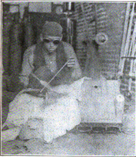
FIG. 2—METHOD OF COVERING, HEATING AND WELDING
