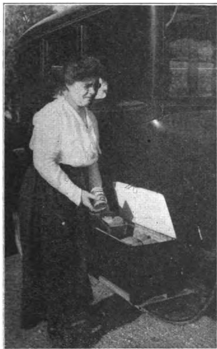
FIG. —THE "EATS" ARE COOKED IN THIS FIRELESS COOKER FROM THE HEAT THROWN OFF BY THE EXHAUST PIPE WITH WHICH IT IS CONNECTED
