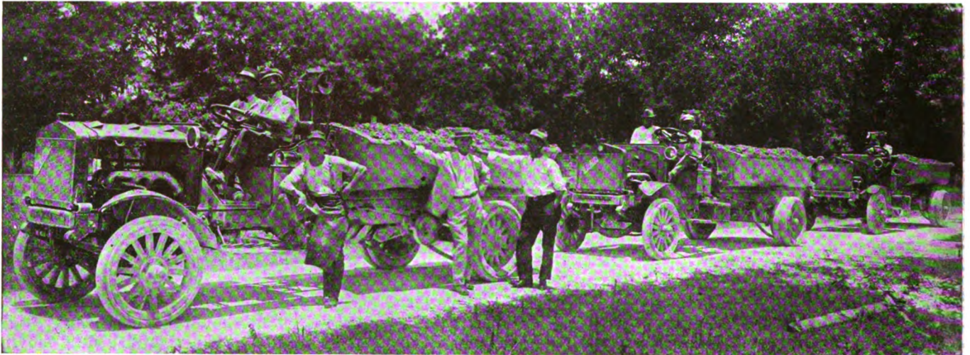
MOTOR TRUCKS EQUIPPED WITH HYDRAULIC HOISTS FOR EASE IN HANDLING ROAD BUILDING MATERIALS. THE HOIST IS LOCATED DIRECTLY BEHIND THE DRIVER'S SEAT.
