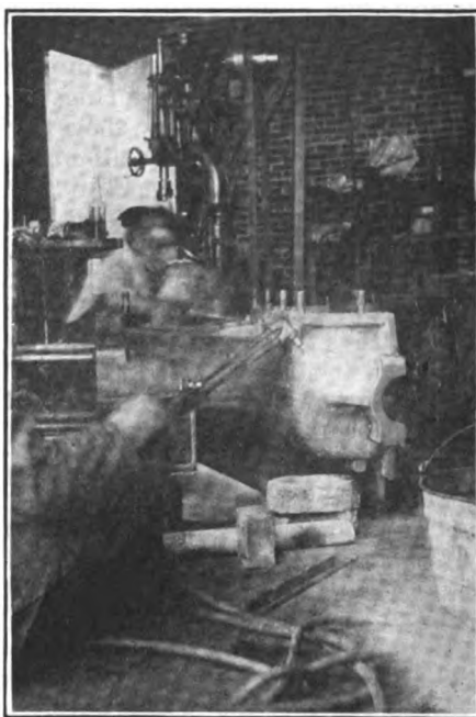
Fig. 2. FINISHING THE SECOND HALF OF THE BEARING WELD
