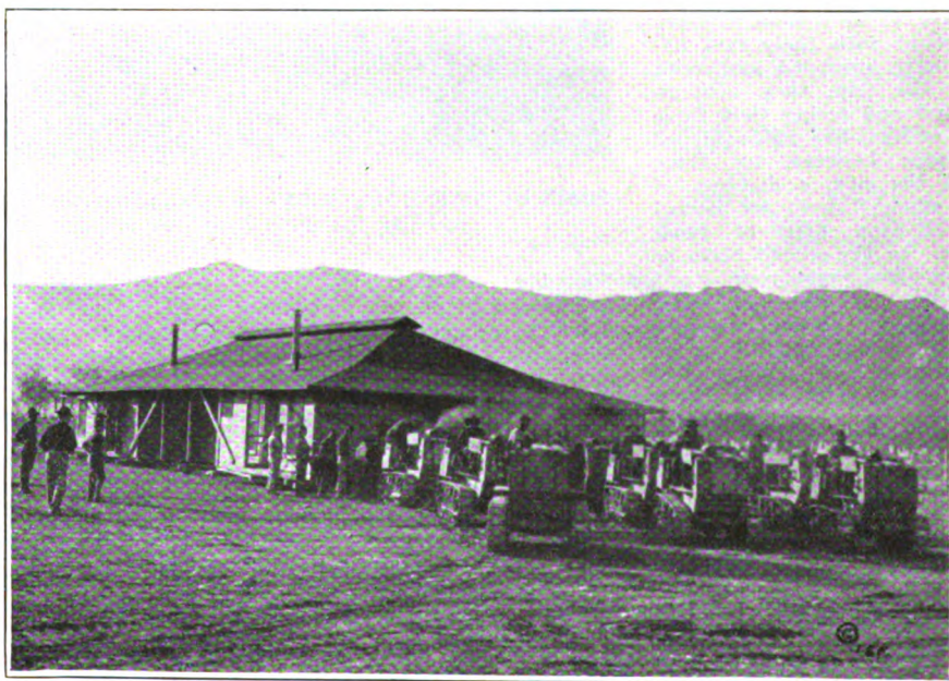
THIS IS INDEED AN INOVATION IN THE MANNER OF MOVING BUILDINGS. THE TANKS WHICH EFFECTED THIS LONG DISTANCE HAUL SAW CONSIDERABLE SERVICE IN FRANCE
