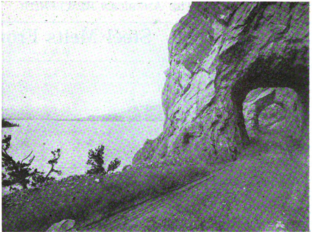
THE WATER RESERVOIR ROAD AND TWIN TUNNELS IN WYOMING
