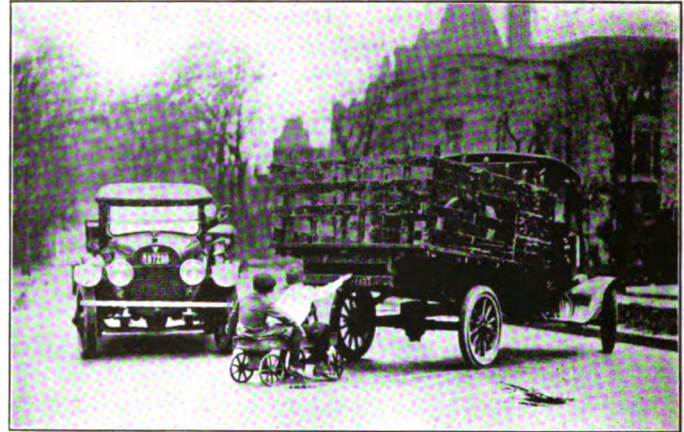
Fig. 6. THE DANGEROUS HABIT OF "HOOKING ON"
