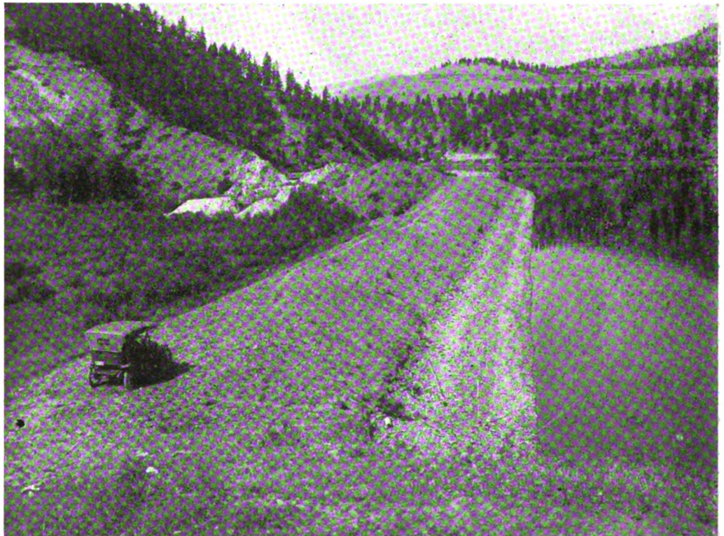
THE CROSSING AT THE CONCONNALLY DAM IN THE STATE OF WASHINGTON
