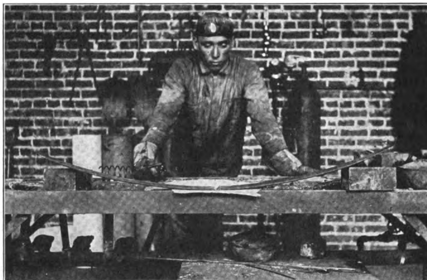
FIG. 1—SHOWING THE ALIGNMENT OF THE BROKEN LEAF
