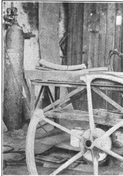
FIG. 1. SHOWING THE LOCATION AND EXTENT OF THE DAMAGE. THE BROKEN RIM IS SHOWN WEDGED UP FOR THE FIRST WELD
