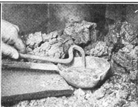
FIG. 9—THE HEATED METAL IS STIRRED TO INSURE A UNIFORM COMPOSITION
