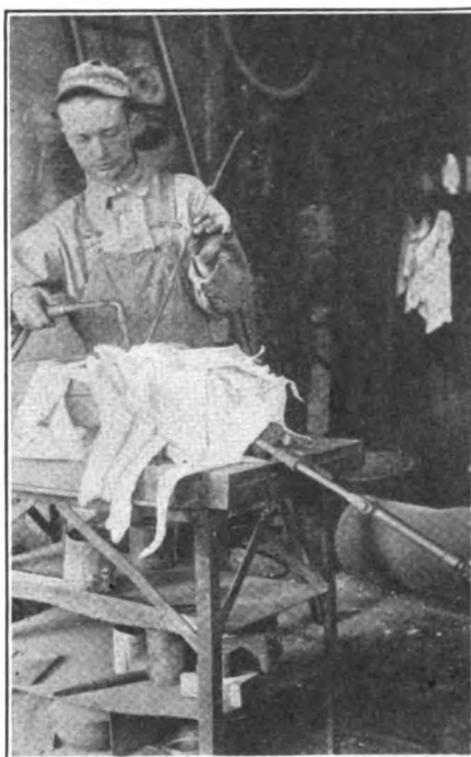
Figure 3. THE ASBESTOS COVERING TO RETAIN THE HEAT
