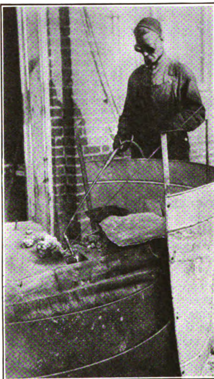
FIGURE 4. STARTING THE WELD
