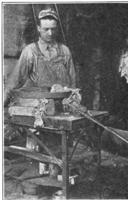
Figure 2. THE ARRANGEMENT FOR CONFINING THE HEAT TO ONE SECTION OF THE RIM
