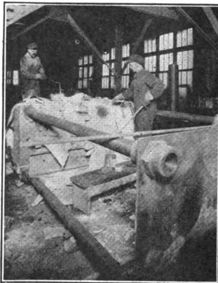
THE BASE IN COURSE OF THE WELDING OPERATION.
