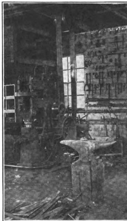
THE INTERIOR OF MR. SNYDER'S SHOP SHOWING A "HOME MADE" POWER HAMMER
