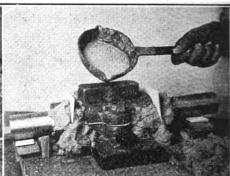
FIG. 10—ONE OF THE SECRETS OF GOOD BEARINGS IS THE MANNER OF POURING
