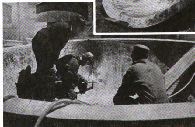
ER WITH A FLANGE ONE FOOT WIDE. BOTTOM — THE FLANGE WAS THREE INCHES THICK AND THE WALLS INCREASED IN THICKNESS TO FIVE INCHES AT THE BOTTOM. THE CUT WAS SEVENTEEN FEET LONG
