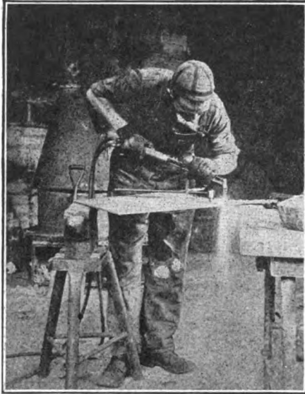
Fig. 2. USING THE ATTACHMENT THAT PERMITS ACCURATE CIRCLES TO BE CUT
