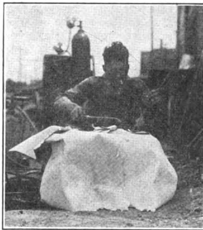
FIG. 3—THE ASBESTOS SHEETS HELD THE HEAT IN WHILE APPLYING THE TORCH.
