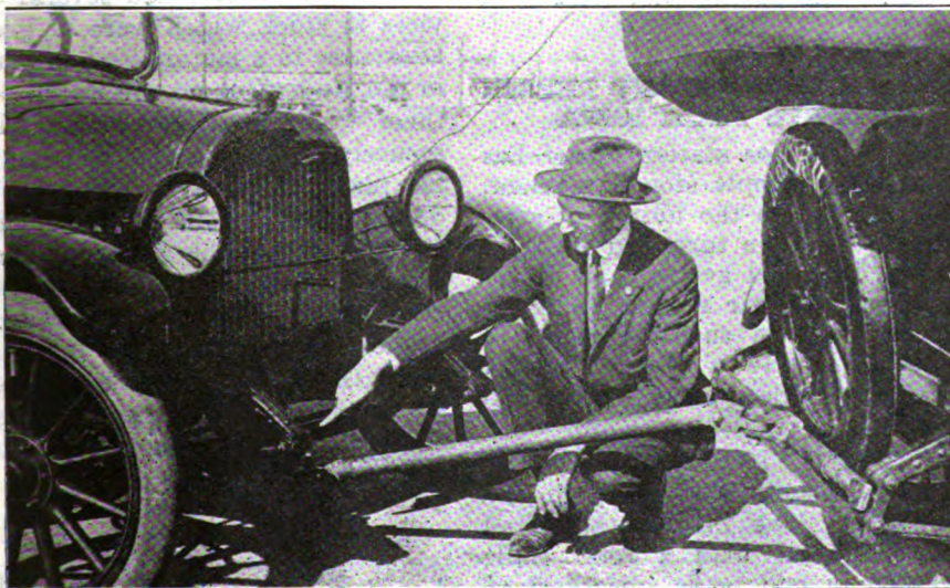
THE DEVICE FOR CONNECTING CARS SO THAT THEY WILL TRACK PROPERLY.
