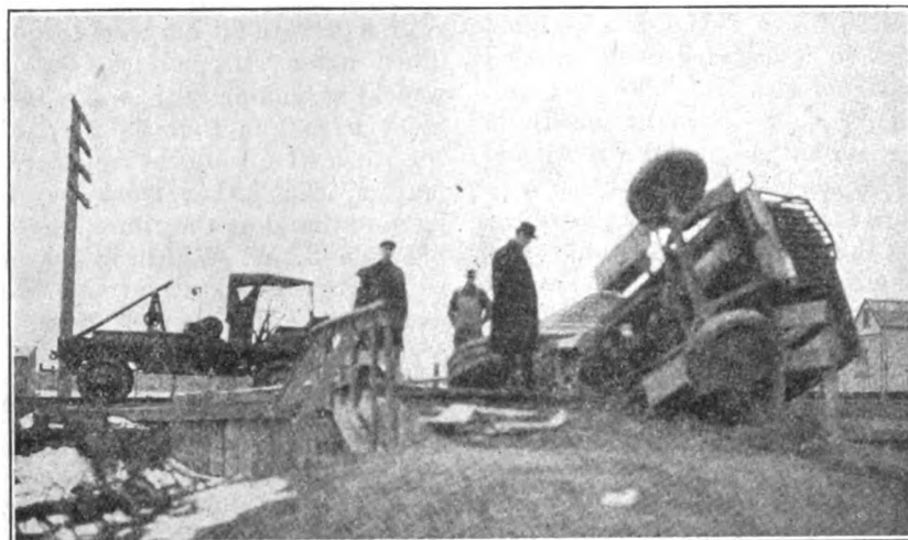
THIS FIVE-TON TRUCK DID MORE DAMAGE TO THE BRIDGE THAN TO ITSELF
