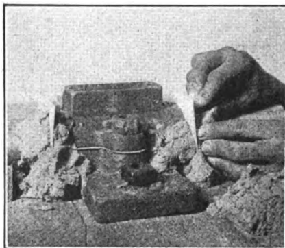
FIG. 7—IT IS GOOD PRACTICE TO CLAMP THE TOP CAP INTO PLACE
