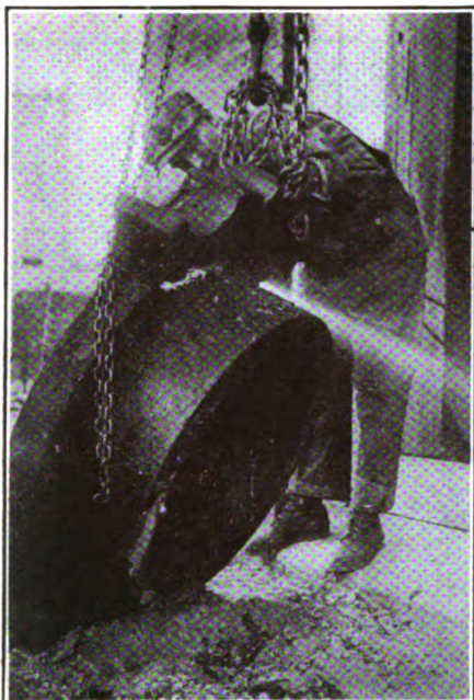
FIGURE 1. GROOVING THE CRACK WITH THE CUTTING TORCH
