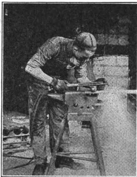
Fig. 1. A ROLLER GUIDE FACILITATES STRAIGHT CUTTING
