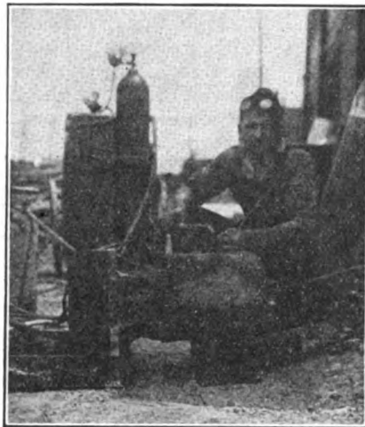
FIG. 2.—THE NEXT DETAIL WAS THE PREHEATING OF THE JOB
