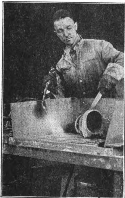
FIG. 3.—FINISHING THE WELD WHILE HOT SAVES TIME AND LABOR—AN OLD FILE IS WELL SUITED FOR THIS SCRAPING
