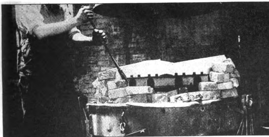
FIG. 4.—THE WELDING POSITION OF THE BLOCK WITH FRACTURE UPWARD
