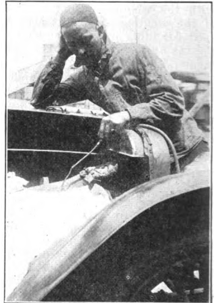
THE OILY PARTS OF THE MOTOR ARE PROTECTED WITH SHEET ASBESTOS
