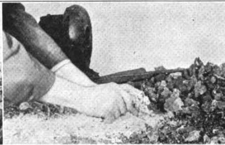
FIG. 2—SHAVINGS AND OILY WASTE ARE FIRED IN THE HOLE
