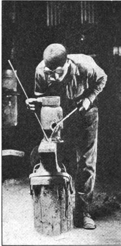
FIG. 4—THE ANVIL TOP CAN ALSO BE USED AS A LEVELING PLATE FOR ALIGNING SMALL JOBS
